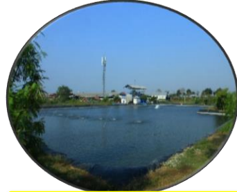
Water Treatment Plant (WTP)
