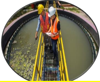
Waste Water Treatment Plant (WWTP)
