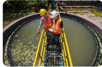
Waste Water Treatment Plant (WTP)
