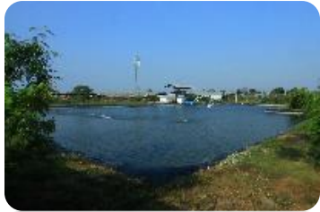
Water Treatment Plant (WTP)
